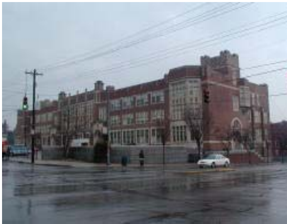
Figure 17 - Heberle School -Vacant Building
